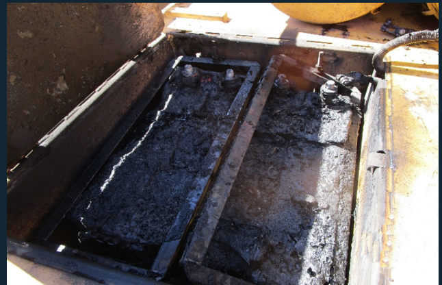
Battery fire. Image sourced from Resources Safety and Health Queensland.
