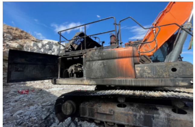
Build-up of combustibles in excavator engine bay causing fire at an open cut quarry. New South Wales Resources Regulator Fires on Mobile Plant, October to December 2021.
