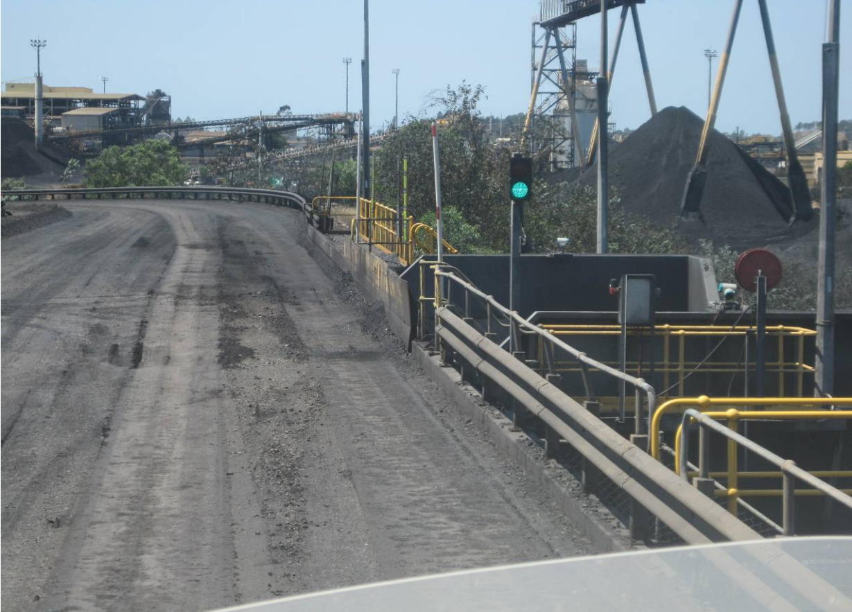
Figure 36 - A well maintained dumpstation is free of tyre damaging conditions such as loose steel-work or rocks
