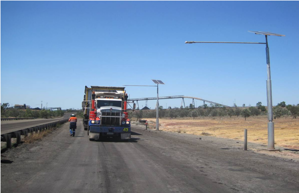
Figure 38 – Vehicle, tyre and rim checking station – note solar lighting
